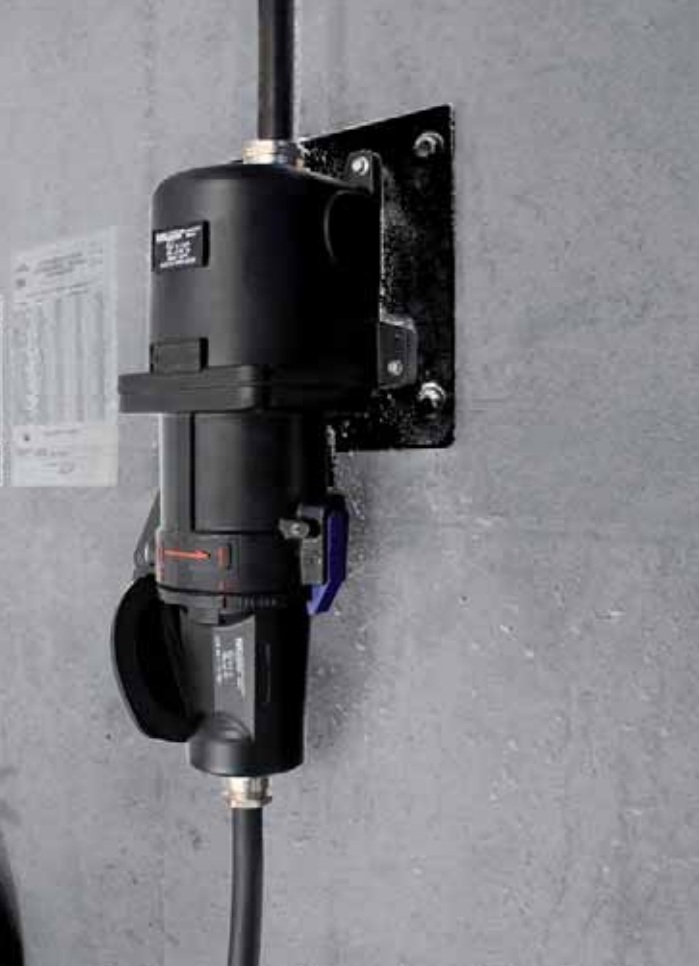
Locking with Allen key
