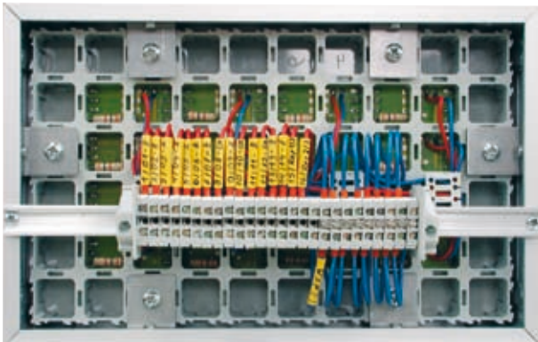
Signalling box designed for mounting in the control desk
