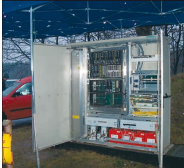
Cabinet before extension
