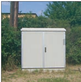
Cabinet before extension
